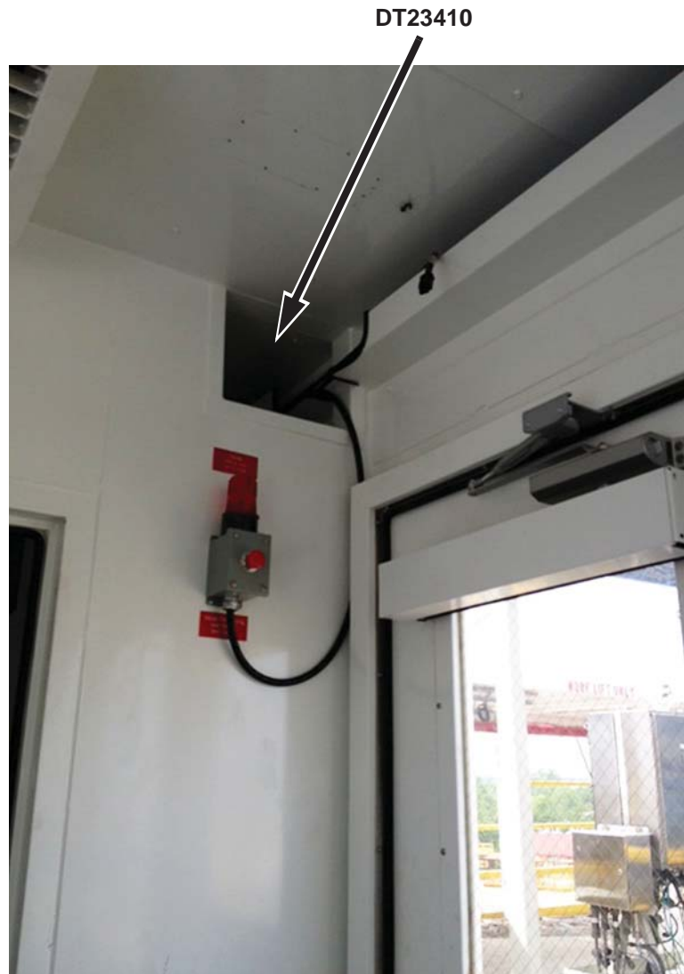
Figure 3: Location for Cover Plate (Canrig P/N: DT23410)
