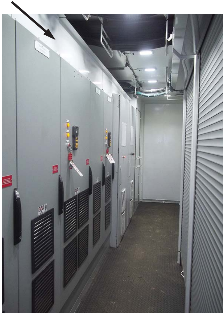
Figure 1: Driller's Cabin Existing Cabinet Cover Plates
